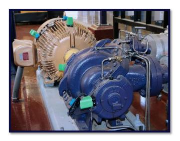
Everactive batteryless sensors continuously stream data to the cloud, providing a 24/7 alarming service for early-warning fault detection.
